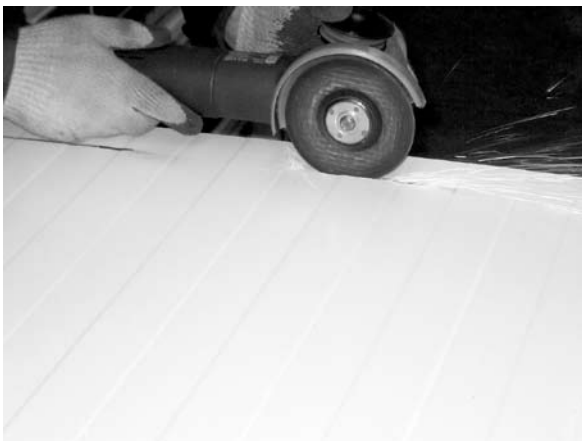
Pic. 2. Do not cut panels with angular grinding machine as anticorrosive covers can be devastated.
