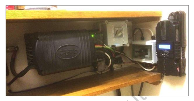
The Outback VFX 3kW inverter and Midnite Classic 250 V charge controller are on the inside of the wall. Again, the battery cables (and fuse) are visible on the left of the photo.
