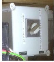
A rotary changeover switch can be used to run the house directly from the generator supply in the event of an inverter failure.
