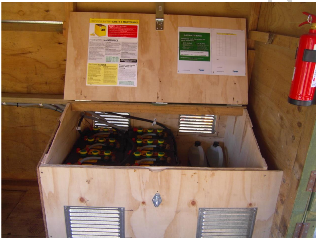
Vented battery enclosure – keep locked
