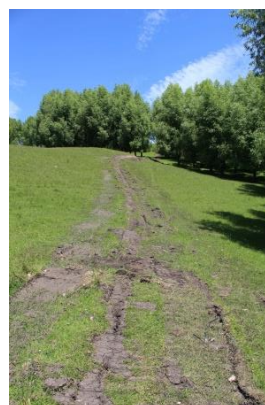
1850m of pipe laid with a pipe ripper in 1 day
