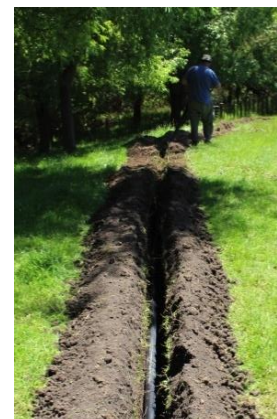
1850m of pipe laid with a pipe ripper in 1 day
