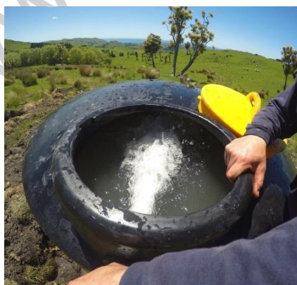
Pressure break tank
